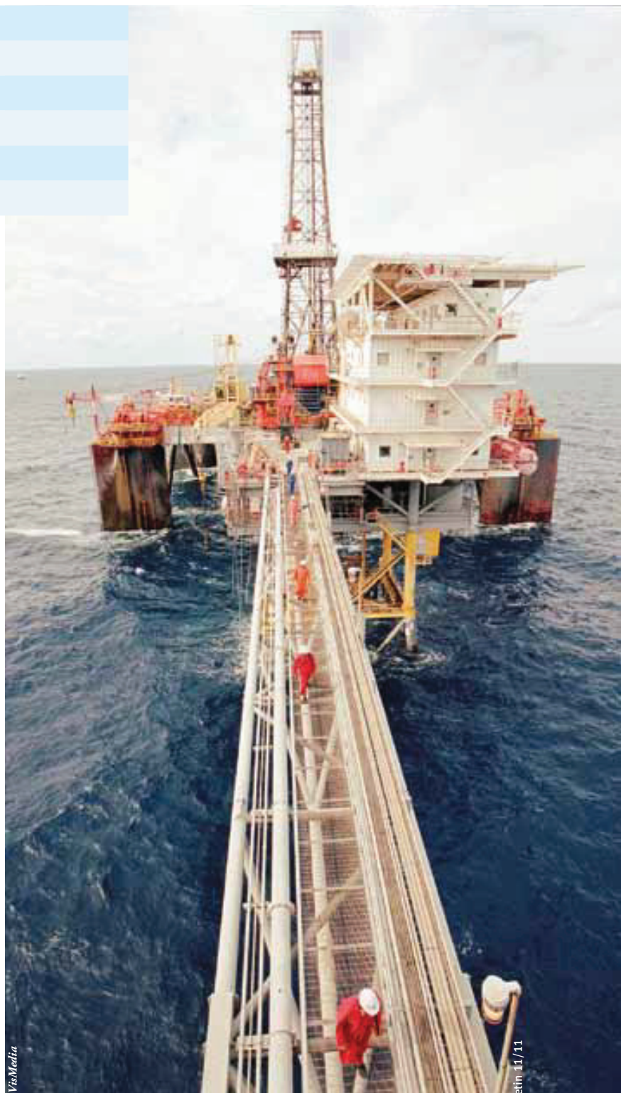
A BG gas installation.
